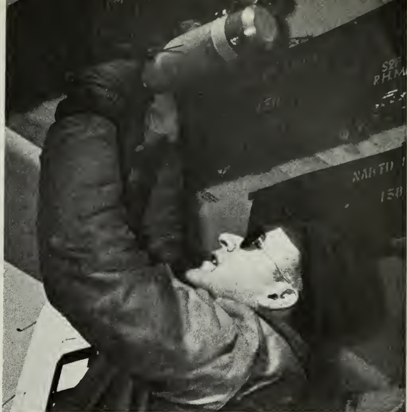
RESERVE CREWMEN work behind scenes to keep their planes on the prowl. Above: AO installs practice depth bomb. Below: Plane's wiring is checked.
